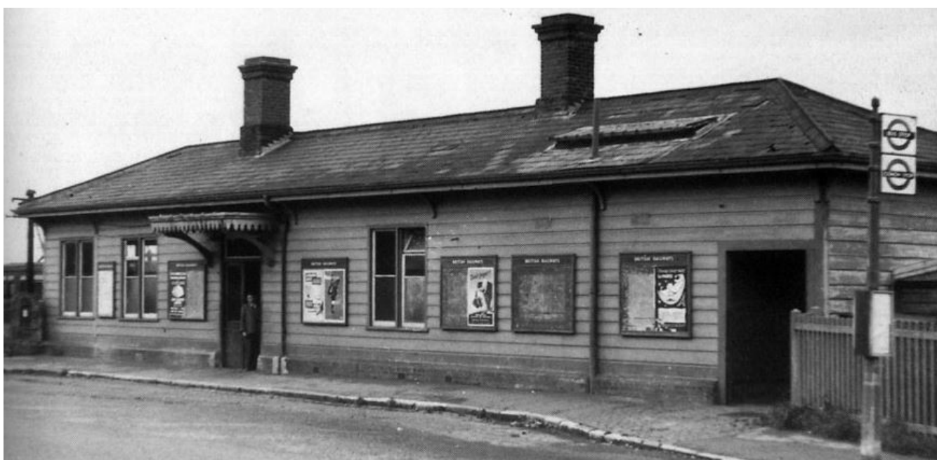
Fig 73 Westerham station on London Road, now demolished (Source: Westerham Heritage Archive)
