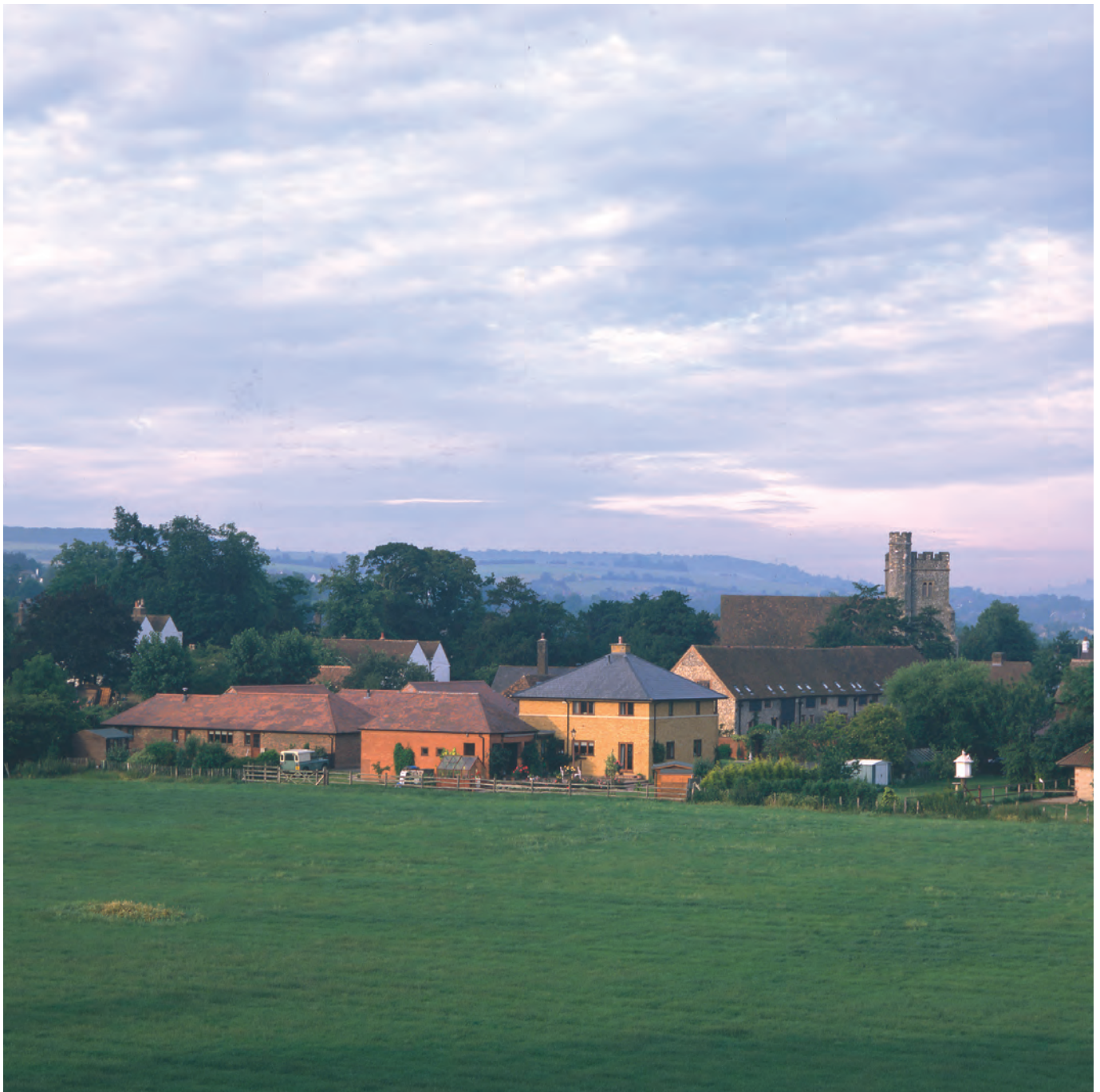
Fig 62 Farningham Mill scheme which combined restoration and new build elements successfully
